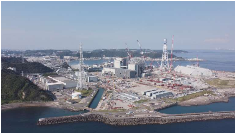
Yokosuka power plant under construction (Kanagawa Prefecture, Japan, photo Sept. 24, 2021)
